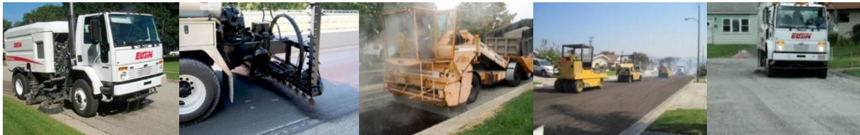
**Phase 2:** Contractors will return with equipment to place a mixture of polymer-modified asphalt emulsion, crushed aggregate, mineral fillers, water, and additives also referred to as asphalt slurry. The mixture is properly proportioned, mixed, and uniformly spread over the prepared street surface. After
